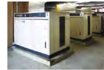
Installation example: manufacturing plant Three SAS55SD units are operated using a multi-unit control system.
